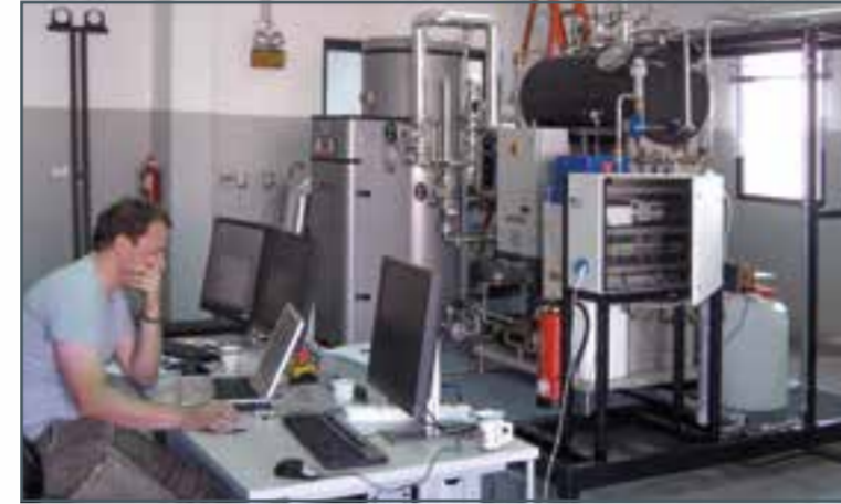
Setting up the control panel
