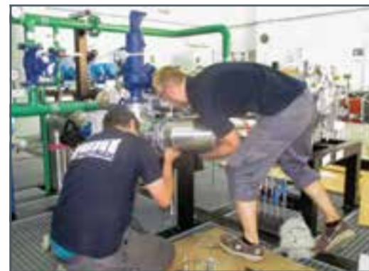
Assembly of the centrifugal pump on site
