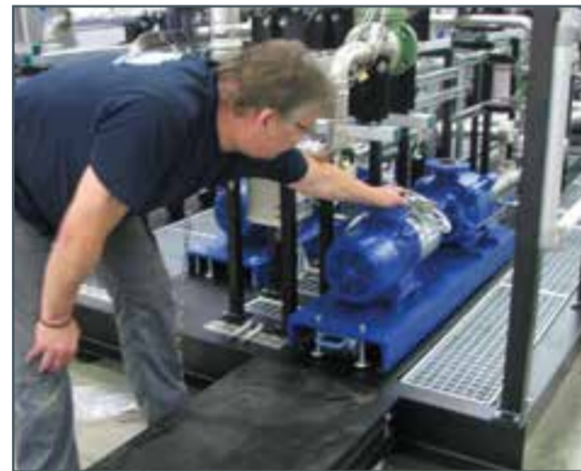
Pumps can be removed and tested
