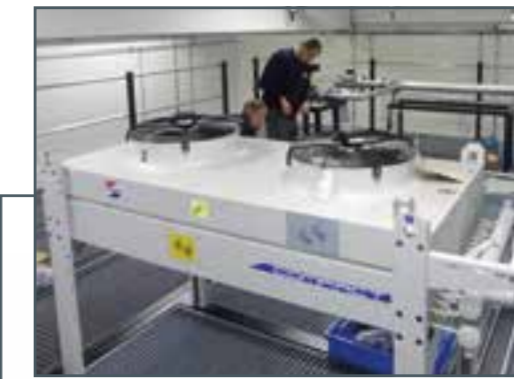
Dry cooling tower
