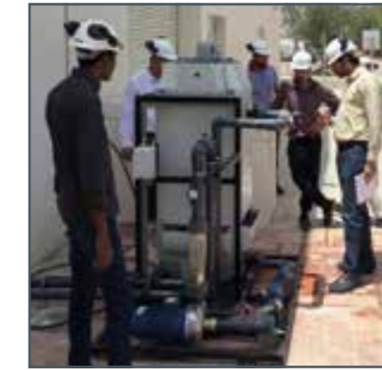
Inspection of the plant on site
