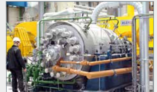
Boiler feed pump of a power station
