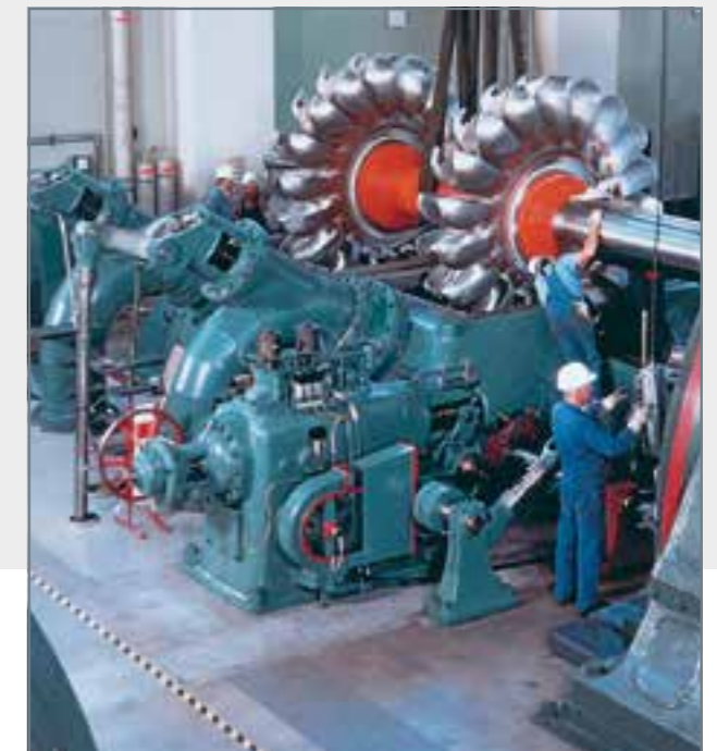
Using a Pelton turbine in a power station
