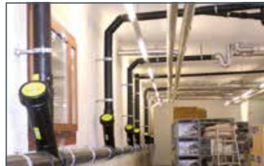
Wastewater engineering in a large building
