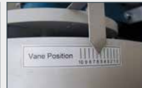
Position of the guide vanes in the Francis turbine
