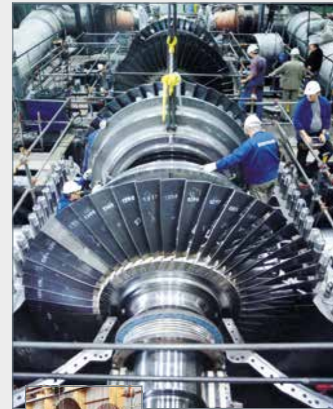
Assembling a steam turbine
